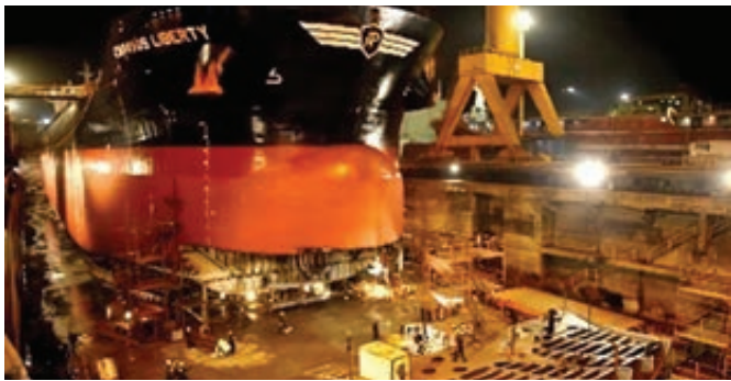
Figure 05 MV Caravos Liberty with extensive steel renewals
