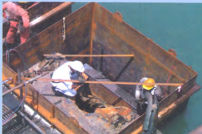
The repair on the damaged Mat being carried out after placing the Cofferdams to isolate the damaged area from the water
