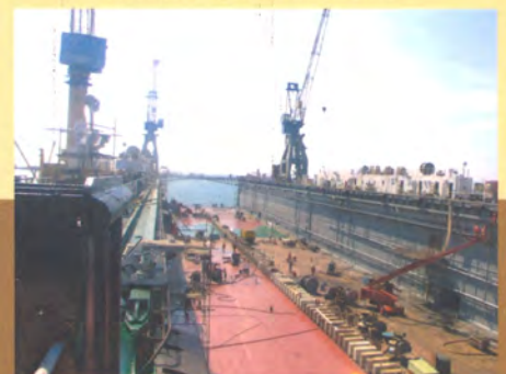
Repairs in Progress
