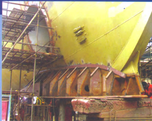
Multi beam eco sounder installaton in progress
