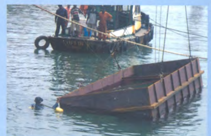
The Cofferd Dam being shifted into place with the assistance of Divers
