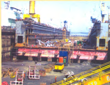
Repairs in full swing
