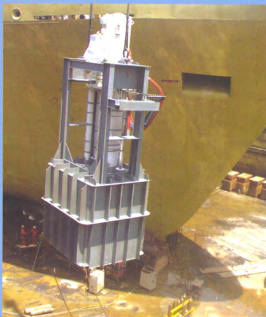
Installation of Retractable Azimuth hruster unit in progress
