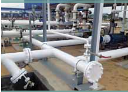
LPG and fire water pipeline for new pump house at Kerawalapitiya LPG terminal for Litro Gas Ltd.
