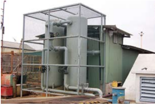
The Compressed Air System near Dry Dock 04
