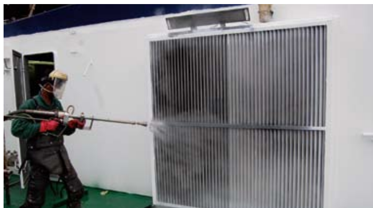
Environment Friendly Hydro Blasting Process in Place
