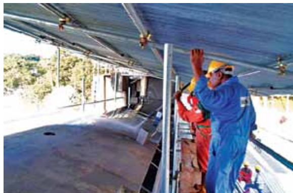
Blasting and painting of spillway gates at Polgolla Dam
