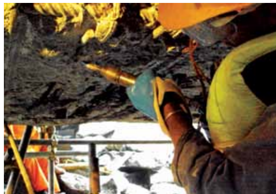
Concrete demolition for crane beam repair work SAGT
